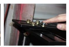
H. Once secure use 3-1 3/4 bolts and 3-WA-1001D spacers to mount the pump to the bracket.
