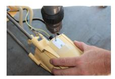
**M.** Install TC-1001 onto fuel tank module, be sure to apply red Loctite onto mounting screws and set screws. Install DT-1002 into TC-1001 using supplied set screws, and adjust 1"- 11/2" from bottom of tank module.
