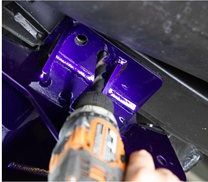
Figure 4: Drilling Bottom Side of Frame
