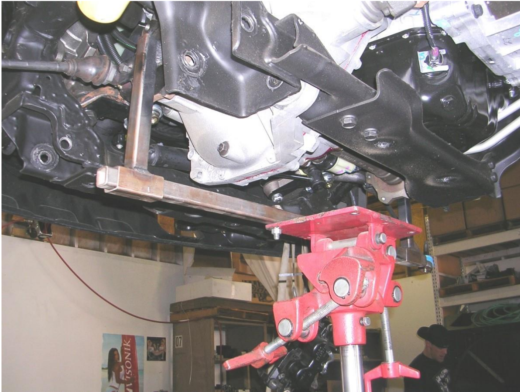
Figure 12: Supporting the front differential before cutting the frame.
