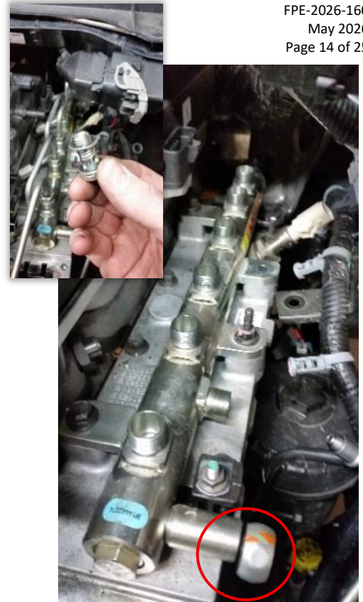
Figure 16: Injection lines removed, fuel return line circled.
