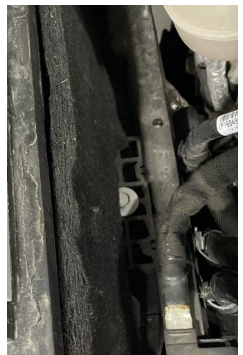
Figure 11: Battery hold down and 10MM retaining bolt.
