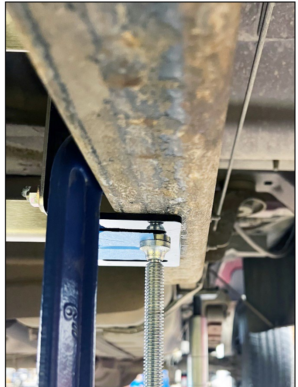
INSIDE / BRACKET EXTENDED AWAY FROM FRAME
