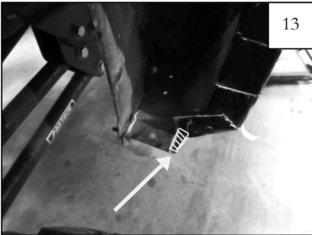
Using a Sawsall, cut off outlined area.
