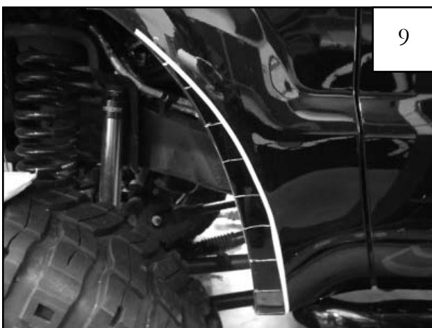
Mark fender with grease pencil about every 2" up to edge of masking tape.
