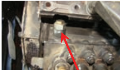
Figure 46 Return Line From the P-7100 Pump
