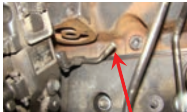
Figure 47 End of steel line from the P-7100 that connects to the tank return line.
