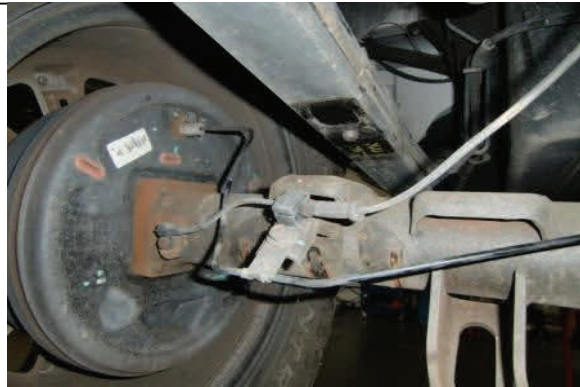
Carefully lower axle enough to install new block
