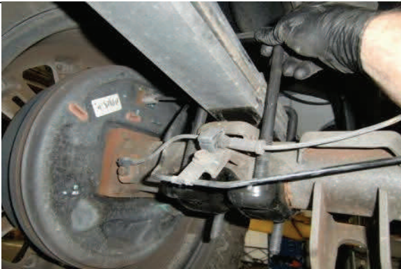
Remove u-bolts and axle mounting plate
